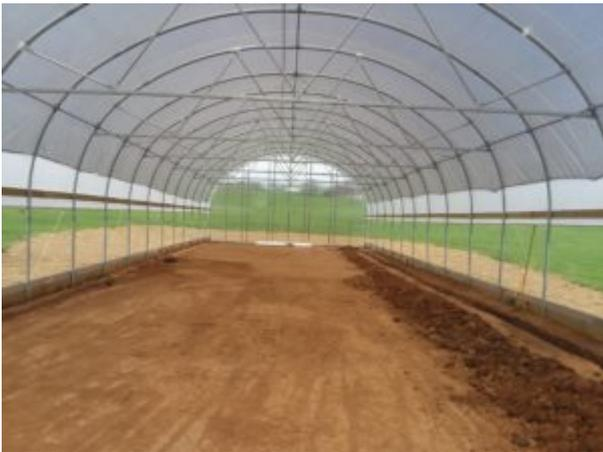
The trench has been dug and is about 18" deep at the far end and 24" deep where it exits the greenhouse at the near end. It was dug by hand because the trench is pretty close to the wall. Digging was fairly easy because half of the dirt was moved into place during site preparation. There was a section about 15' long that was a pain to dig because there was a lot of 1" to 3" gravel in the ground.
