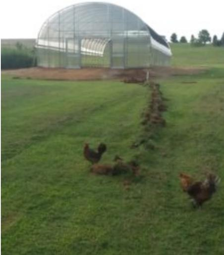
Looking north from about 100' from the greenhouse you can see the trench that was started with a subsoiler and finished by hand with a trenching shovel. I was going to rent a trencher but the digging was fairly easy at this point so I decided to dig it myself (*issue #1*). It ended up taking about 3 days of intermittent digging to get the trench run, the pipe laid, and to make the hookup to the well.
