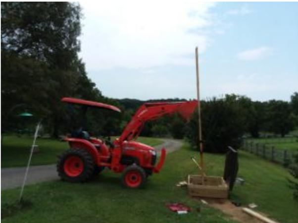
I used the bucket of the Kubota to pull the pipe, wire, and well pump up from a depth of over 220'. The old pipe was 2" schedule 80, 20' pipe with threaded metal connectors that weighed a ton. It took half a day to put it to the surface and take the pump off. The pump was a 3 HP, 17 A monster(!).
